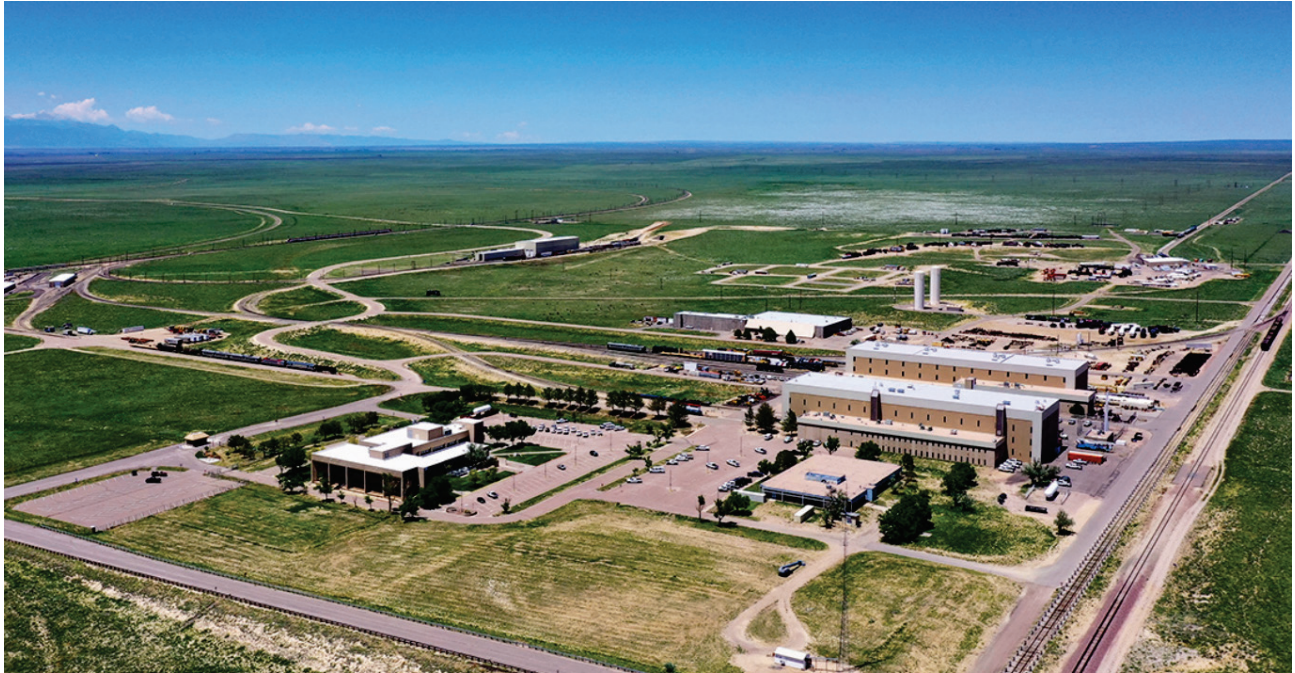
Figure 6.11 Federal Railroad Administration Transportation Technology Center (Pueblo, CO)
